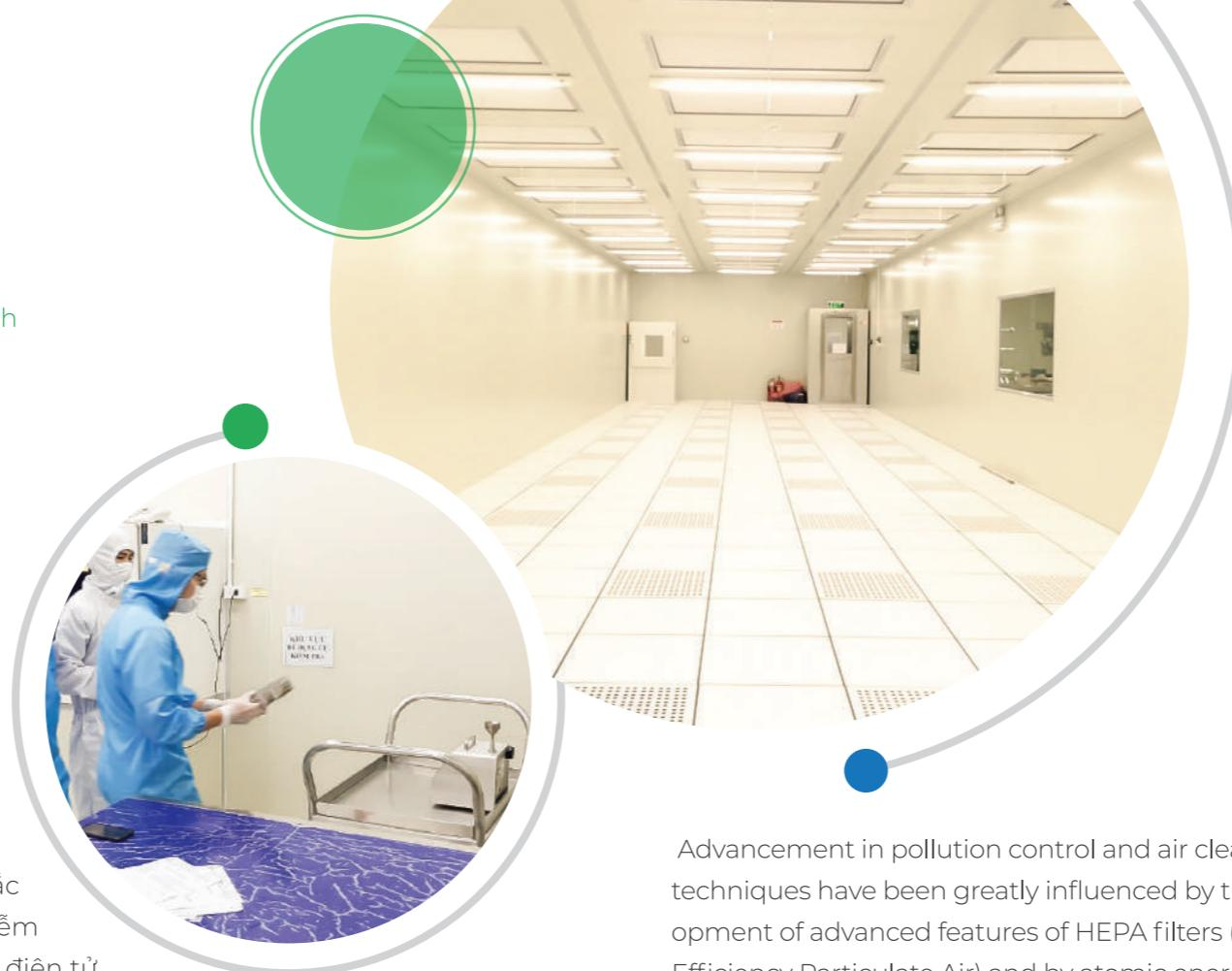
**Clean room (Clean Room - CR)** according to international standard ISO 14644-1 is defined as [Room to control concentration of floating dust, construction design maximum limits dust accumulation, super small dust particles arising; simultaneously controls other necessary factors such as temperature, humidity, pressure ..]
